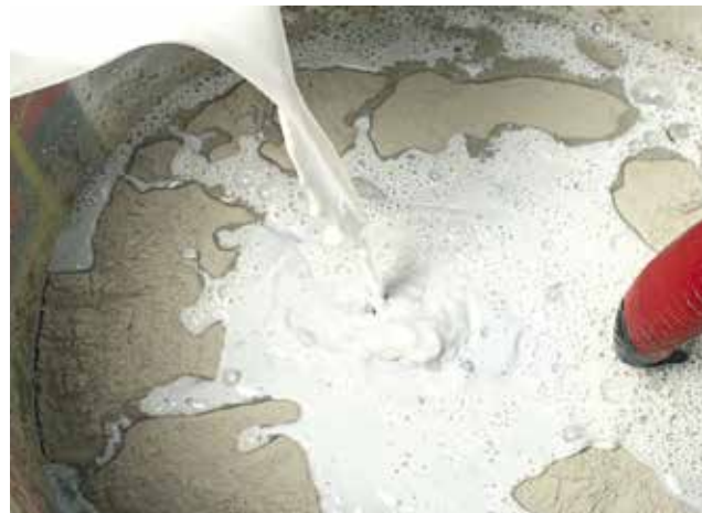
Adding to mixing water.
